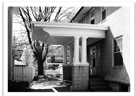
Restored porte cochere at 1612 22 nd Street
