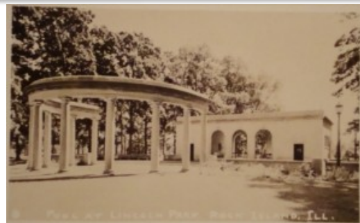
Early View of Pool House and Peristyle, RockIslandPreservation.org
